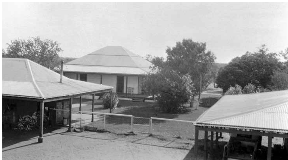
Strelley Station in 1948 (Battye Library, SLWA 112512PD)
