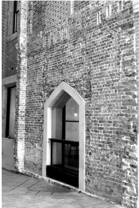
Original brickwork. (Richard Offen)
