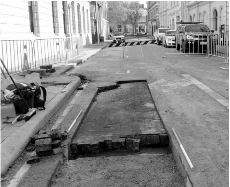
Mouat Street looking north from High Street, showing one of the sections of wooden street found during the pipes replacement program (courtesy Archae-Aus).
