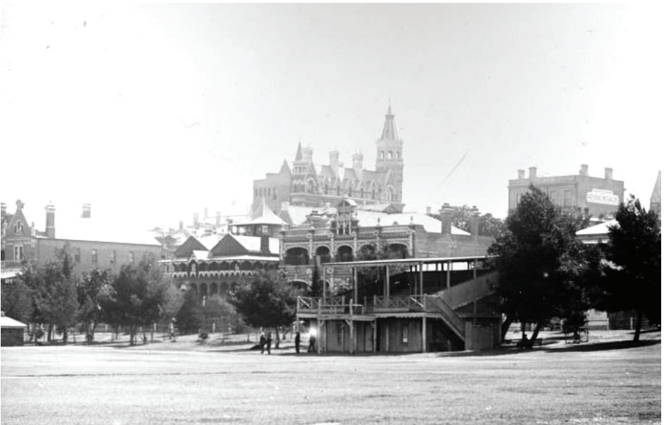
Small grandstand on the Esplanade, Bazaar Terrace in the background, 1906-1907. (Courtesy Battye Library, SLWA 207332PD.)
