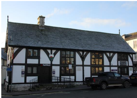
The bank building where the Quarter Sessions took place
