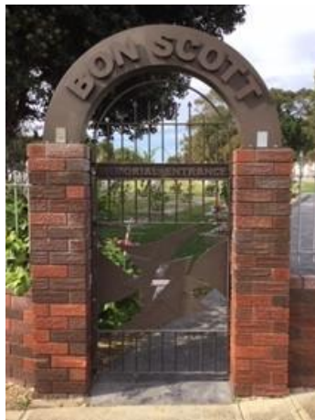
Bon Scott Memorial Entrance Gate, Fremantle Cemetery Photo: Heather Campbell
