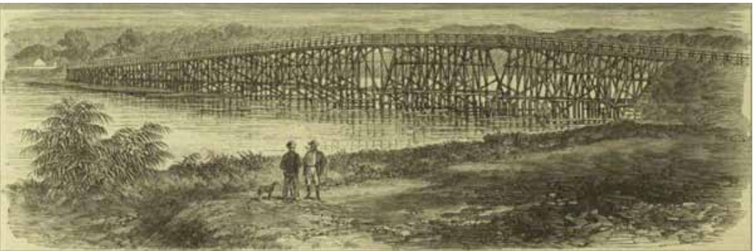
Bridge at North Fremantle, Western Australia.
