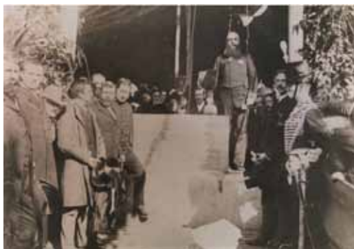
Governor Broome laying the foundation stone of the Victoria Public Library St Georges Terrace 20 June 1887.
