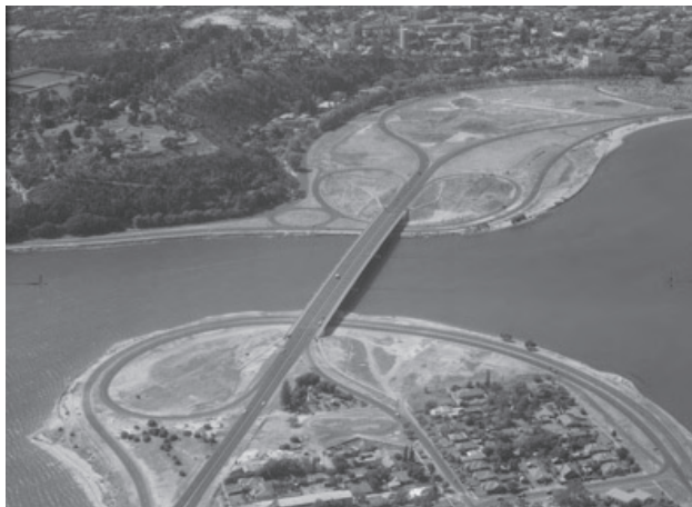
Aerial photograph of the Narrows Bridge and freeway construction.
